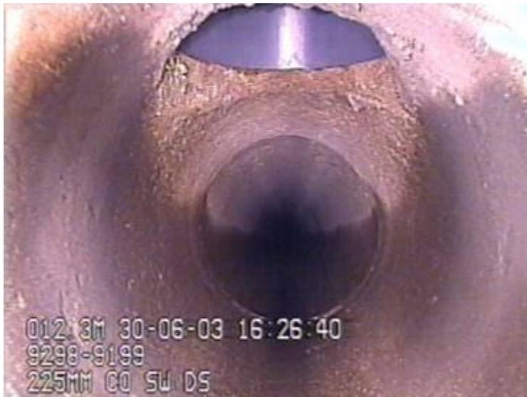
A: Connection- A connection at 12 O'clock with defects and is in service
