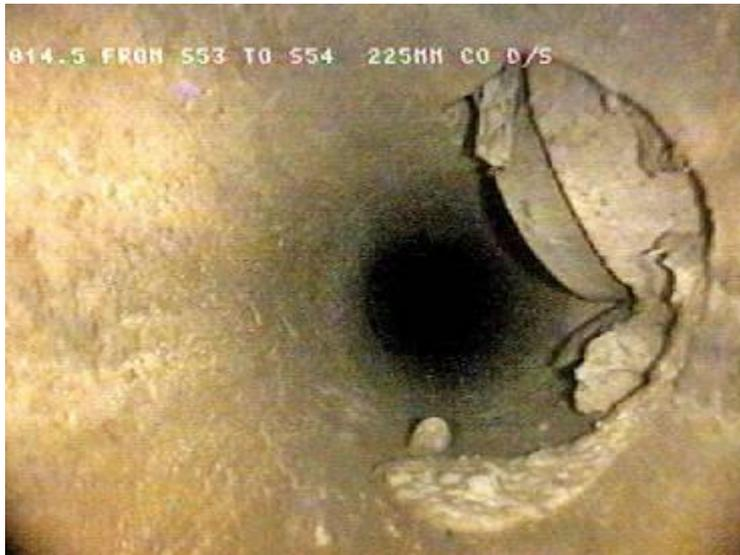
B: Connection Defective- A connection intruding into the main pipe at 2 O'clock
