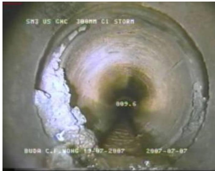
A: Deposit Attached- Foul material from the sewage attached to the inner wall of the pipe
