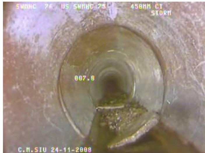
B: Deposit Settled- Coarse material deposits at the bottom of the pipe
