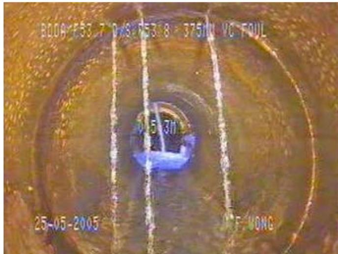
D: Infiltration- Groundwater running continuously through faulty joint
