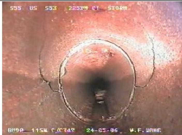
D: Circumferential Fracture from 9 to 3 O'clock
