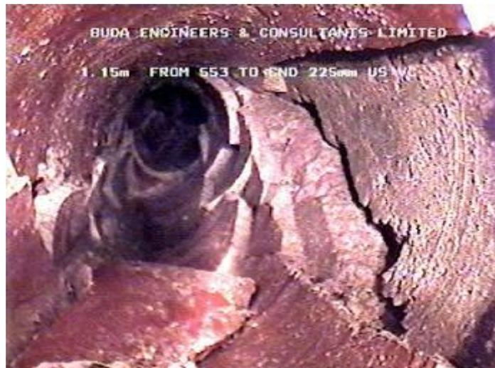
B: Collapse of pipe section with 30% reduction in cross sectional area
