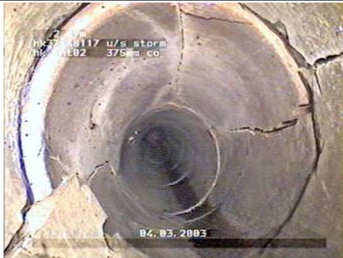
A: Broken- no missing pieces but some have noticeable displacement
