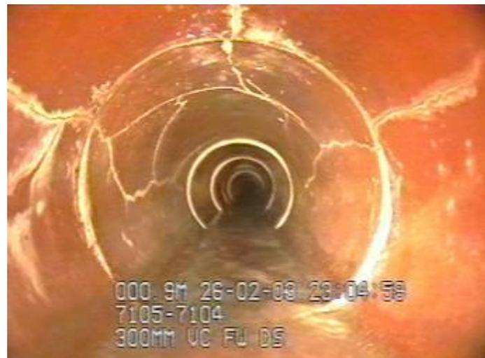
C: Multiple Crack from 9 to 2 O'clock
