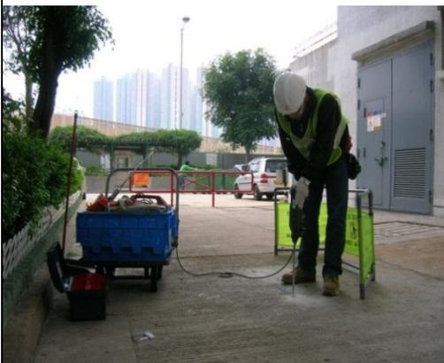
E: Hole drill for gas leakage detection.
